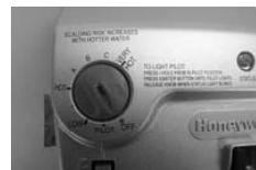
Gas Control shown in the "OFF" position
